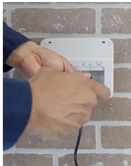
Image 0.13 Securing sensor to backplate
