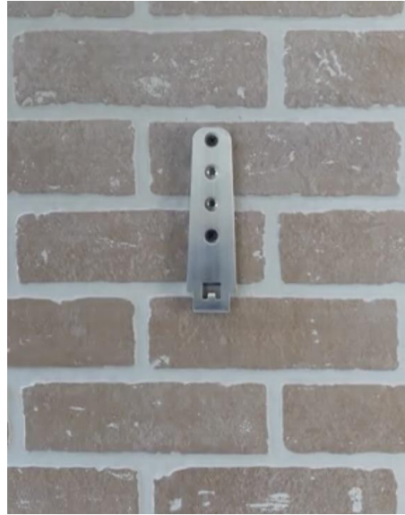
Image 0.4 Final bracket install
