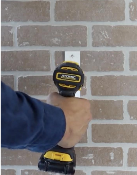
Image 0.3 Pre-drill holes with drill bit
