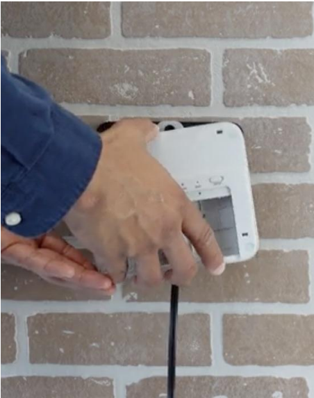
Image 0.11 Attaching sensor to backplate
